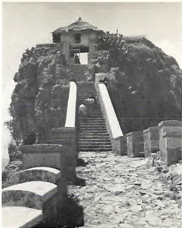
The only gate to the mountain top
